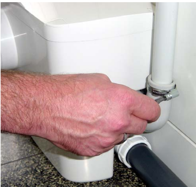
(Pic.4) To connect the pressure hose, please fasten the DN 25 pipe at the outlet bow, which is on the right at the tank of the SEKAMATIK 10 E 6M, with a clip. Install the pressure hose upwards (best way: first vertically, than horizontally) in a loop above the sewer level. This will avoid that waste water will flow back into the tank in case excess water (e.g. heavy rain) is in the sewer. Install the pressure pipe directly to the next soil stack. Please check again all connections and make sure that they are sealed. Now connect the unit with the power cable to the main supply and the unit is ready for operation.
